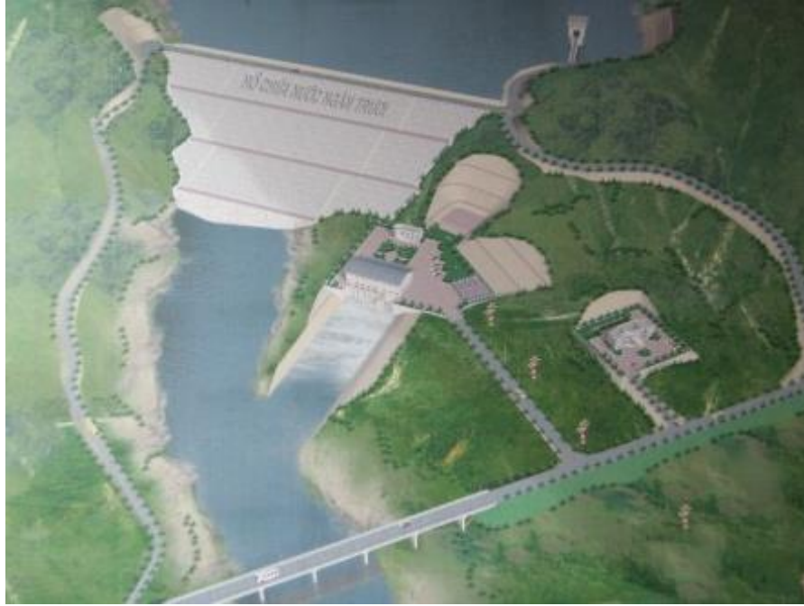
Figure 5.2 Overview of Ngan Truoi reservoir and Cam Trang hydropower dam
