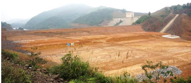
Construction of the Cam Trang dam and spillway
