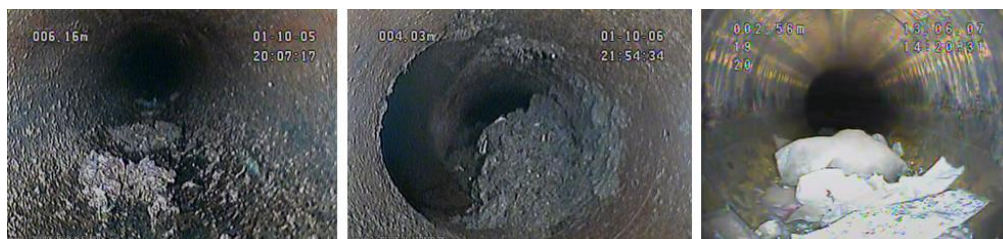
Figure 5 Accumulated waste inside pipeline
